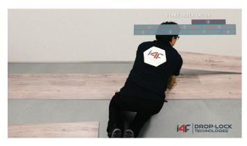
**Remove alignment planks (planks 0 & 3)** Remove planks 0 and 3 by angling them out.
